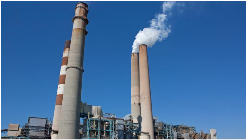
Big Bend Power Station is a major coal-fired power plant near Apollo Beach, Florida.
